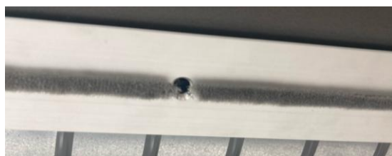
The hole in the bottom rail for the door hook
