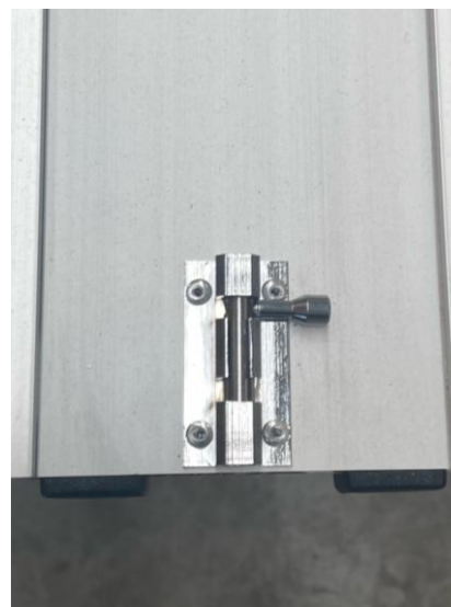
Socket bolt for locking the mullion to the floor
